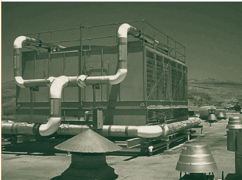
Modified Central Plant Cooling Tower Installation.
